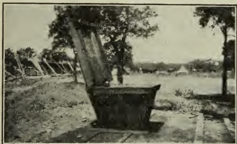
FIG. 44.—Hopper in cover of pit for reception of liquid garbage. It contains a removable burlap sack supported by upturned nails acting as hooks.
